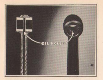
"The wrist pin bushing comes in two halves and we insert them in the connecting rod from each side, being careful that we don't cover the oil hole in the rod."
