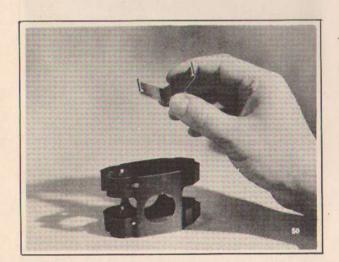
"This small "U" shaped spring is a head stabilizer and is installed in the solid half of the piston opposite the vertical slot to tighten the struts."
