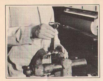
"Now, while you have the pistons disassembled from the rods, Pete, how do the piston pins and bushings look?"
