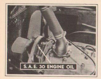
Ed: The water pump bearings take a shot of S.A.E. thirty engine oil at every lubrication. Just add enough oil to make it run out the overflow. And, oh yes . .
