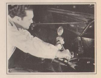
If you use the Tension Indicating Wrench and pull the head nuts down uniformly with a new gasket and plenty of good gasket paste, that's all you can do. Even then, some of the exhaust gas may still get through to form acid. That's why the Eveready Prestone Manual says --
