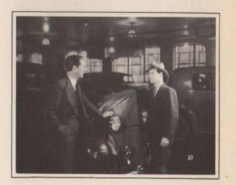
Ed: Here's a One Twenty that we just got started on. Bob has the engine running with a good cleaning solution. He'll run it for about ten minutes at 180 to 200 degrees . .
