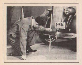
WALT: Work the front of the car up as high as it'll stay and measure the distance from the floor to a referance mark you made on the radiator shell. Be careful to let loose of it slowly, or it'll jolt down and give you a false reading.
