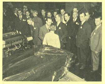
Here the group inspects the aircraft engines being prepared for shipment. Pliofilm bags from which moisture is removed is one of many precautions taken to insure safe shipment of this powerful engine. It is then ready for its trip to aircraft assembly plants.
