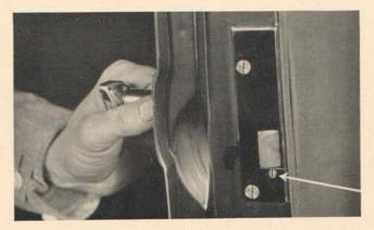
catch up and down, you will find that this condition can be corrected by tightening the adjusting screw. We are locating the screw for you in the attached view.
