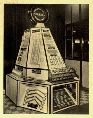
cannot be missed by any customer who comes in. It is a 6-sided affair, 5 sides of which have parts mounted. The framework was made from some old lumber we had in the shop, and the outer part of ordinary plywood sprayed with a coat of aluminum, and trimmed at the corners and edges with black metal moulding.
